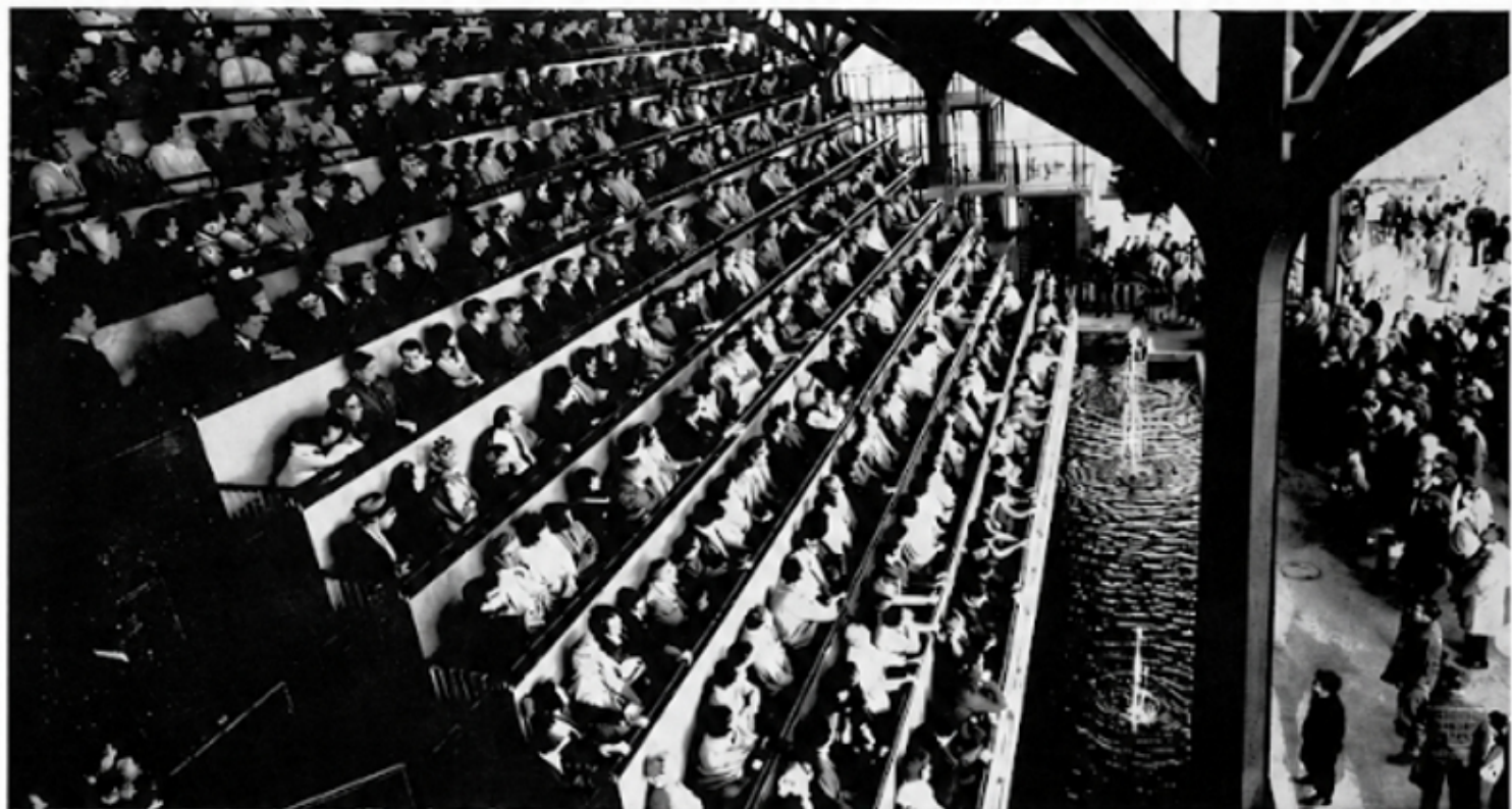
A close-up of the "People Wall" at the IBM Pavilion, New York World's Fair. This grandstand seats 450 persons, approximately 36 tons of people. The audience, seated, is lifted to the auditorium in the dome. After the show, the unit is lowered, the audience leaves and the process is repeated.
