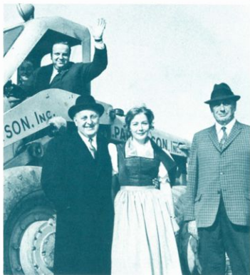
A bulldozer breaks ground for the Pavilion of Austria. Left to right: Commissioner General of Austria, Consul Manfred von Mautner-Markhof (in bulldozer); Governor Charles Poletti, vice president, International Affairs and Exhibits at the Fair; Miss Elfriede Mundl of the Austrian Institute in New York; and Mr. Robert Moses, Fair president.
