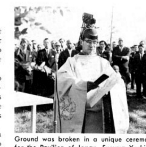
Ground was broken in a unique ceremony for the Pavilion of Japan. Susuma Yoshida, Shinto Priest, performs the Shinto rites of purification prior to the groundbreaking.
